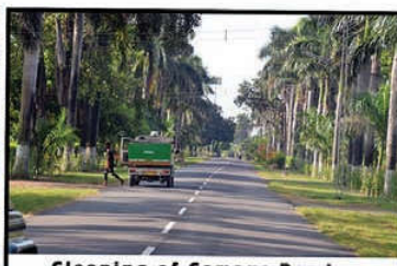
Cleaning of Campus Road
