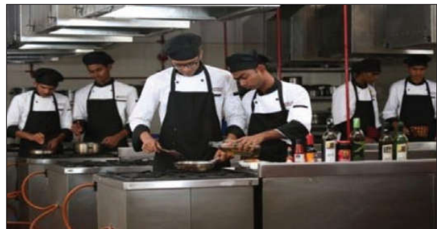
Modern Kitchen cooking area with chimney
